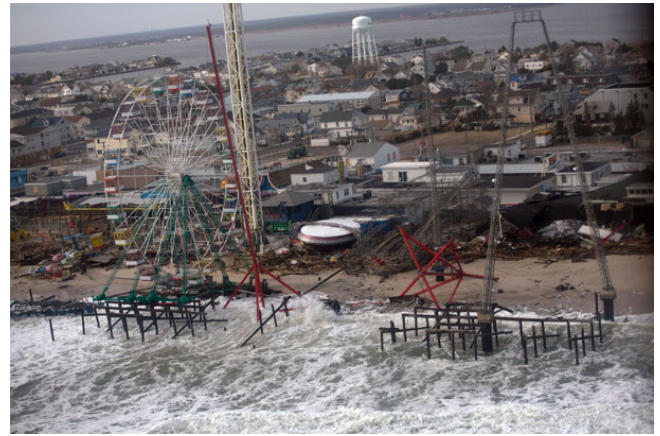
An aerial view of Sandy's strong storm surge that caused extensive damage along New Jersey's barrier beaches.
